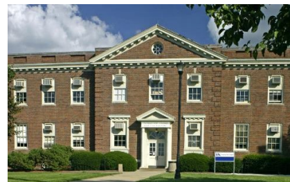
Thomas Poe Cooper Building Forestry and Natural Resources
